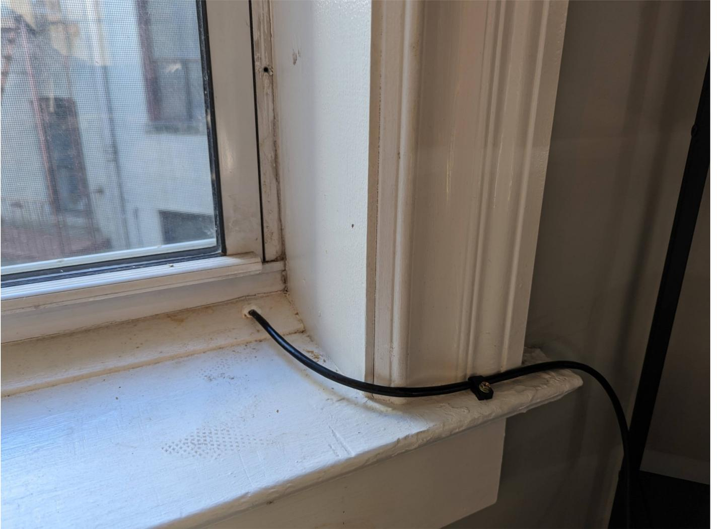
Example of a plastic window with a hollow frame. Was able to drill through the bottom frame of the window which is hollow inside.
